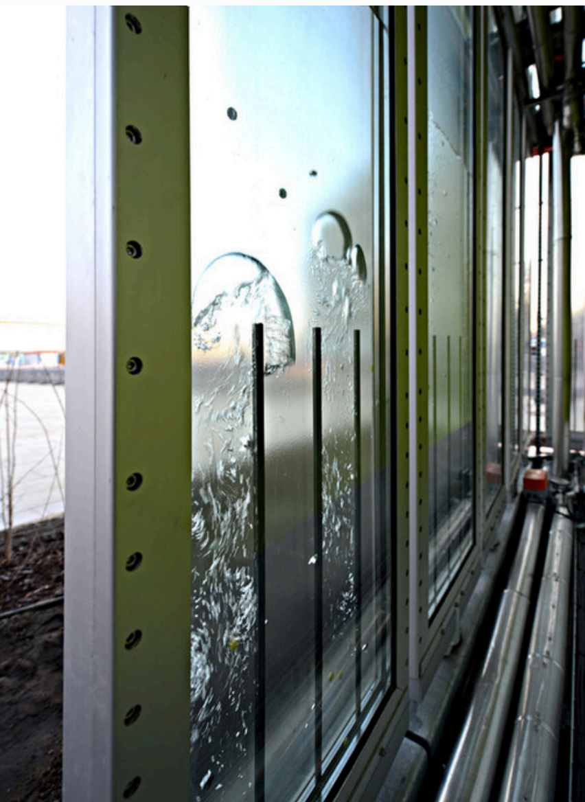
SolarLeaf-Louver viewed from Backside with hidden Horizontal Support System
